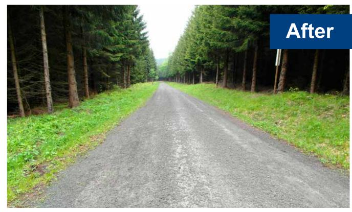
Regular road maintenance using the SWO1 road maintenance equipment will improve the operating life and consevation of the sideways and diagonal profils, ensure better water drainage and combat excessive growth of grass and weeds between te edge of the road and the shoulder.
